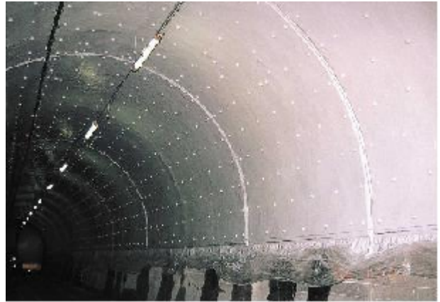
Reinforcement and the scupper of fiber sheet applied tunnel lining
