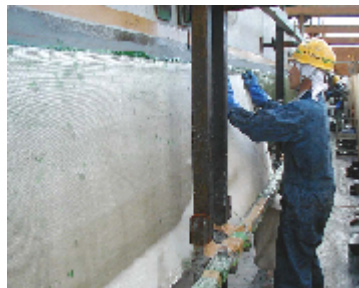
Fiber sheet mounting work ( horizontal beam end )
