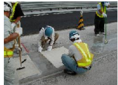
Fiber sheet mounting work ( floor-slab upper surface part )
